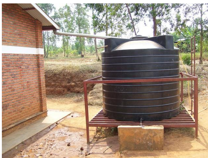
Figure 30: PVC Tank used to collect water during water harvesting operation (Earth Eclipse, 2018)
